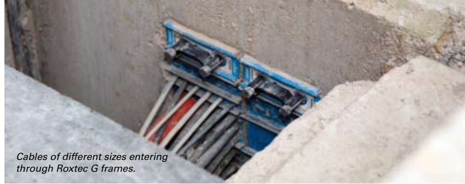
Three sealed cables – and one spare yet to use!
