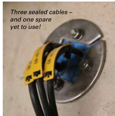
Cables of different sizes entering through Roxtec G frames.
