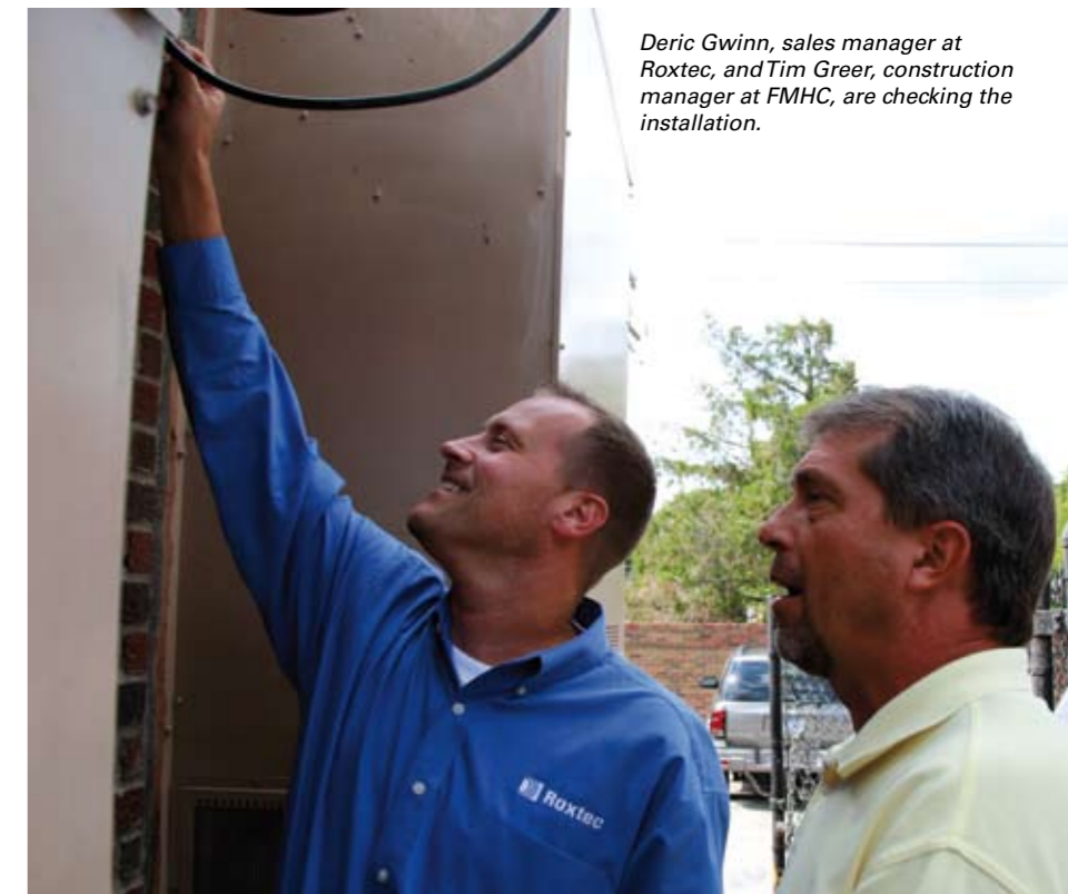
There is still room for more cables to enter the shelter!
