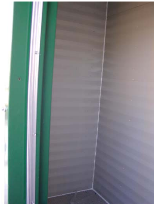
Fig. 12 Walls Showing joints With Caulking
