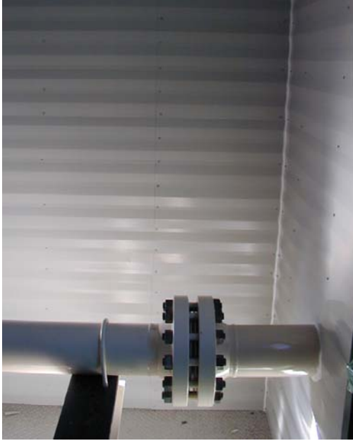
Fig. 13 Pipe Wall Penetration Sealed
