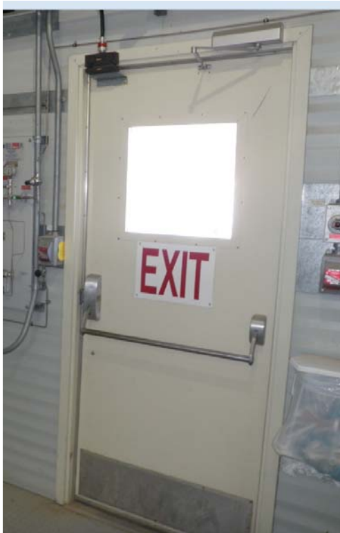
Fig. 14 Self Closing Door with Gasket Seal
