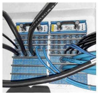
and enabled scalability. In addition, Roxtec seals require minimum maintenance while offering built-in spare capacity. Hiperbaric is using Roxtec S Ex transits for multiple cable penetrations, and Roxtec C RS T Ex seals around single ethernet connections. In the equipment, there are mostly 5mm to 50mm thick electrical cables for sensors and actuators, whereof some armored, but there are also pneumatic tubes.
