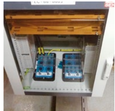
Indoor enclosures in offshore environment. Roxtec has a wide range of solutions available to seal from IP4x to IP67, as well as Ex and EMC versions in different frame materials. This picture shows a Roxtec C KFO, a plastic frame that handles large amount of cables in a small footprint.
