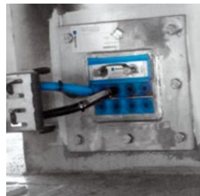
Frames that can be bolted to the structure, like the Roxtec SFHM, are suitable for insulated panels and sandwich or non-weld demand installations.
