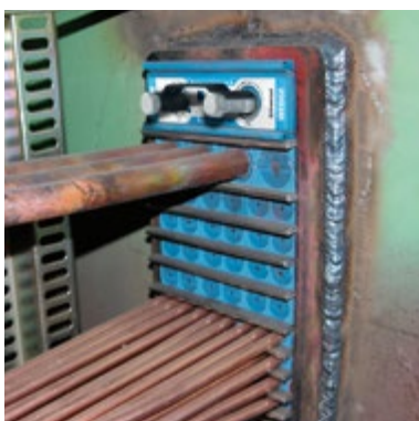
Roxtec S frame – multiple metal pipe penetrations through a single square or rectangular opening in the deck or bulkhead.
