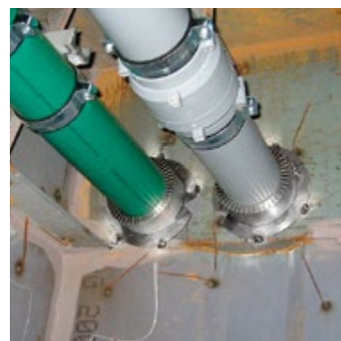
The Roxtec Sleeve-it™ Fire penetration seal is a single side installation solution which protects single plastic pipe penetrations against fire hazards. Its openable aspect specifically benefits retrofit as well as new-build projects.
