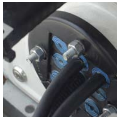
A pre-installed Roxtec ComPlus entry seal is easy to open up later when cables need to be added.
