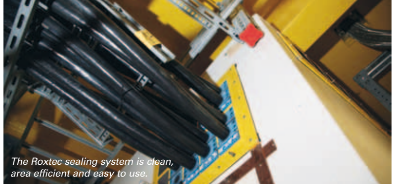
Roxtec seals are adaptable to cable and pipes of different sizes through modules with removable layers.
