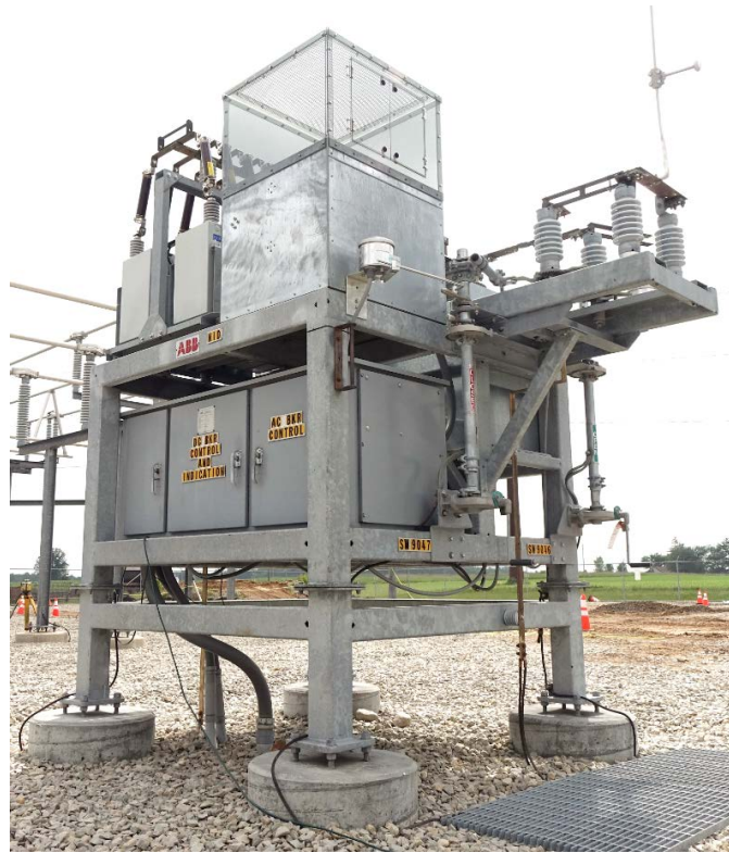
Figure 5-12 Physical representation of a neutral blocking device deployed in the field Courtesy of EMPRIMUS, LLC
