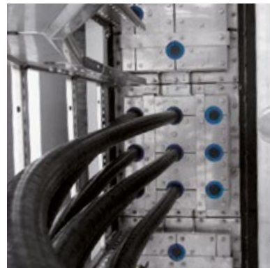
Special Roxtec H frame solutions for large cables
