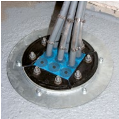
Roxtec R frame in bolted sleeve
