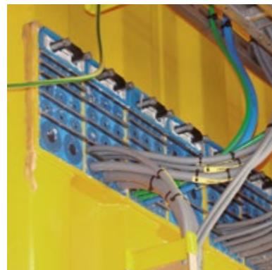
Welded Roxtec S frame
