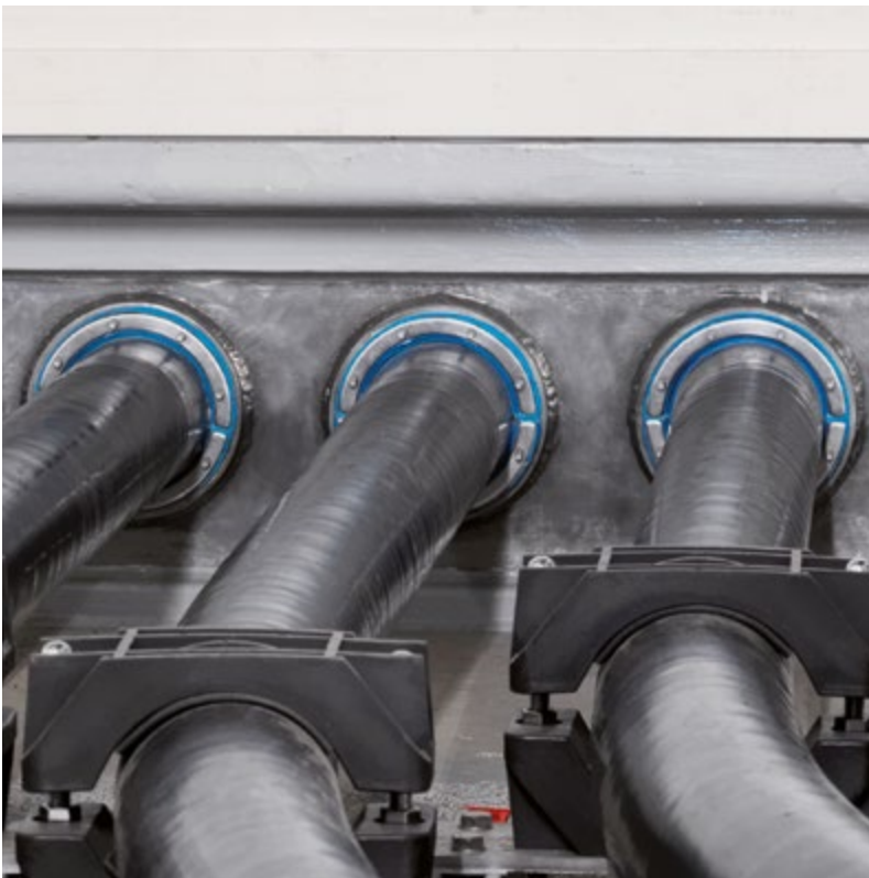
Roxtec RS seals for power cables
