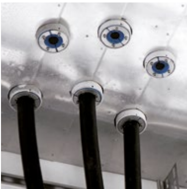
Roxtec RS seals for cables to switchgear
