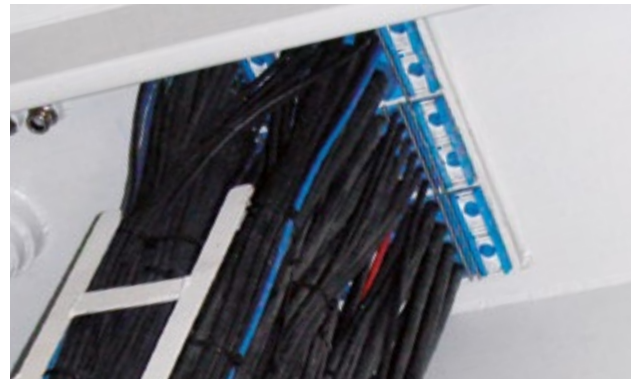
Welded Roxtec S frame
