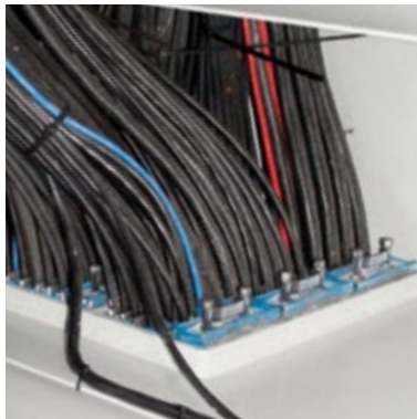
Welded Roxtec S frame
